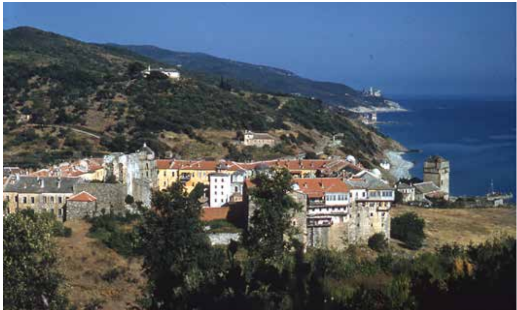
Fig. 9. Iviron Monastery, general view.
