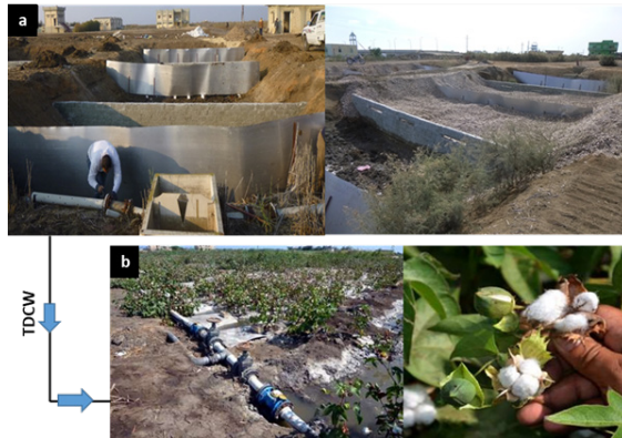
Pilot plant P4 for drainage canal water treatment and reuse: a) setting up of a sequenced hybrid constructed wetland in Lake Manzala in Egypt, b) cotton plants irrigated with treated drainage canal water using gated pipes.
