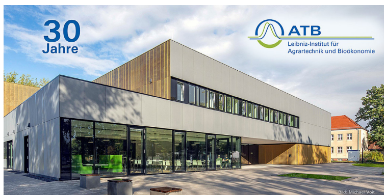
Figure 2: Since 2019, the latest ATB research building CIRCLE has been expanding the infrastructure. CIRCLE stands for 'Center for Research and Communication in a Circular BioEconomy'. With 25 laboratories and 23 offices, the research building offers workplaces for about 60 employees, especially in the fields of microbiology and IT. A 330 m 2 dividable conference room, another two meeting rooms as well as a 125 m 2 cafeteria offer space for knowledge transfer and communication.
