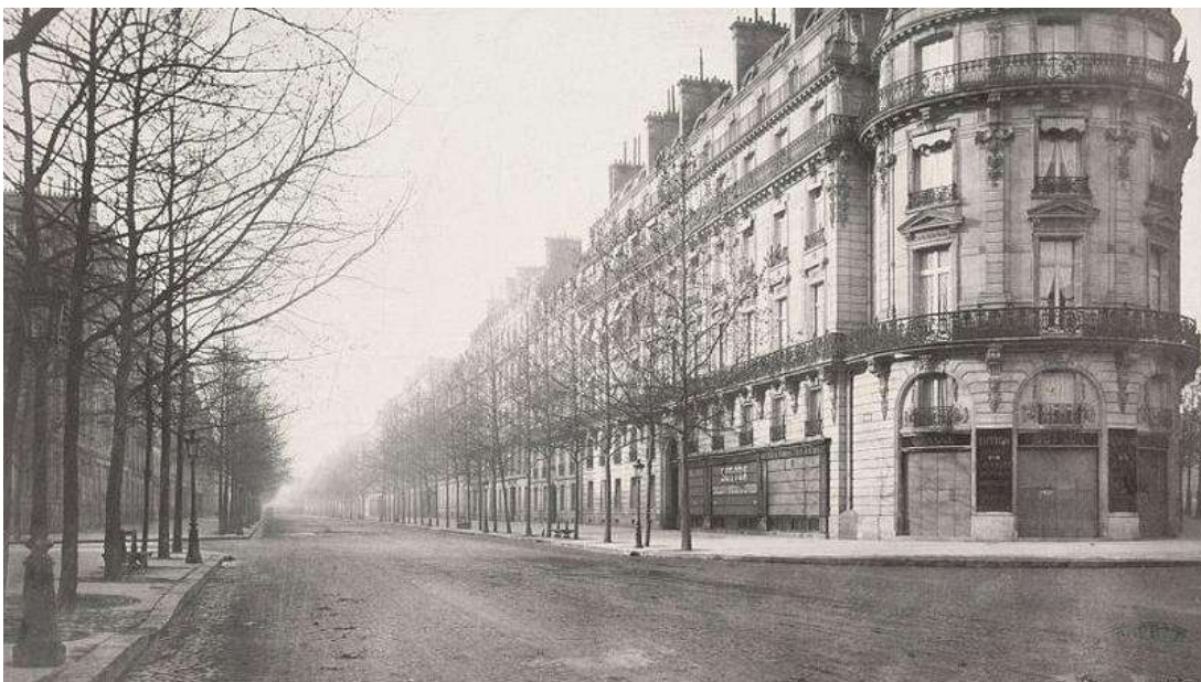
Fig. 4 – C. Marville, Boulevard Haussmann , (post 1857) https://it.m.wikipedia.org/wiki/File:Charles_Marville,_Boulevard_Haussmann,_de_la_rue_Miromesnil,_ca._1853%E2%80%931857.jpg
